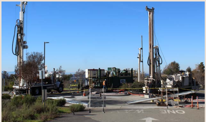
Drill rig equipment drills 400 feet deep
