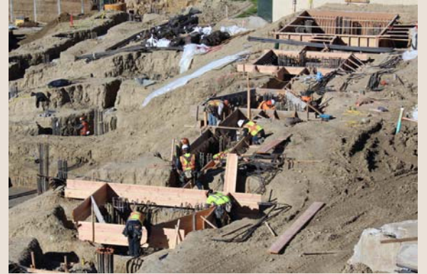
Concrete Footing Installation
