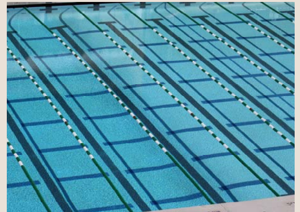
Newly Renovated Pool adjacent to Building 9
