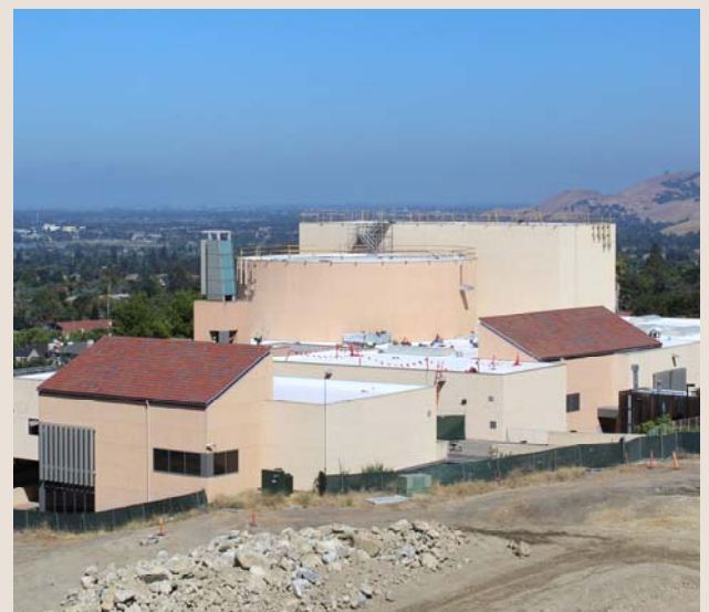
Smith Center Roof Replacement
