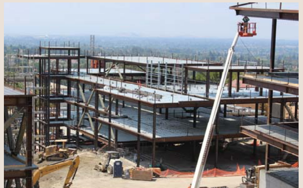
Structural Steel construction at the future Arts Building
