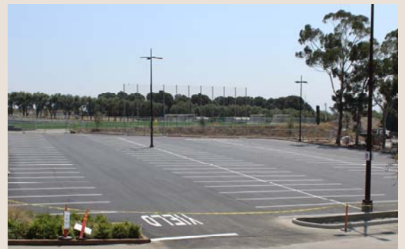
Newly renovated Parking Lot D
