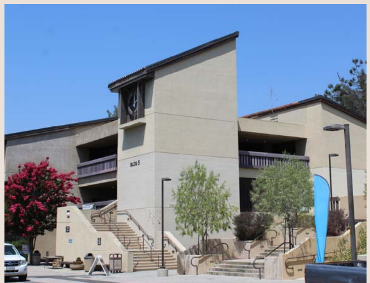
Building 5 will be renovated in 2019
