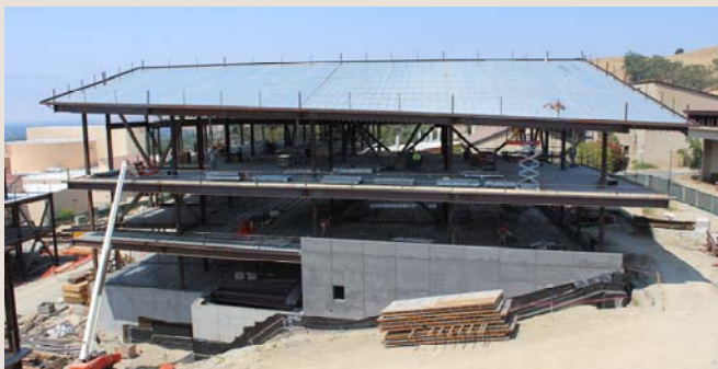
South elevation of the future Learning Center
