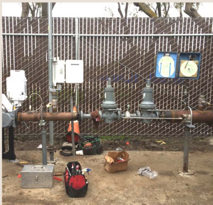
New gas meter main installation
