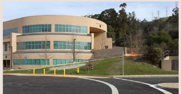
Future stairway path at Building 7 exterior
