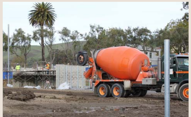
Softball dugout construction
