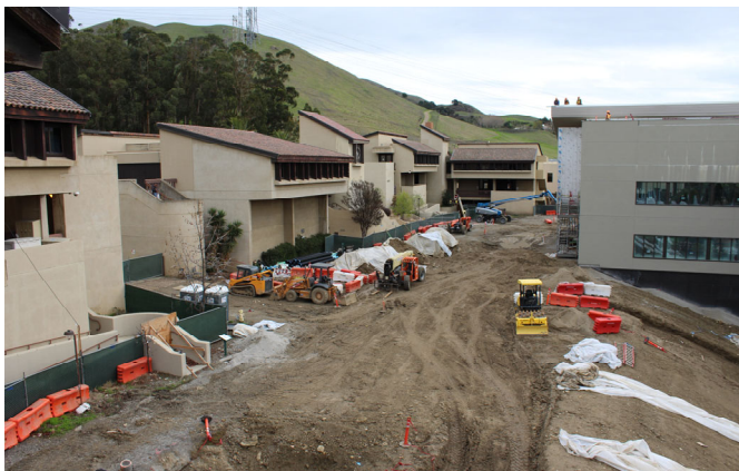
Main Street Site Work
