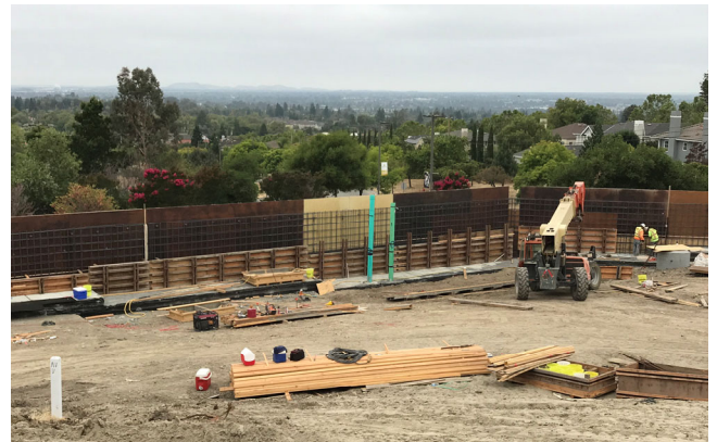
Lot X: Retaining wall forming
