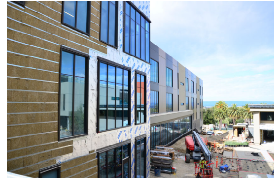
Building 1: north elevation, looking west towards the bay
