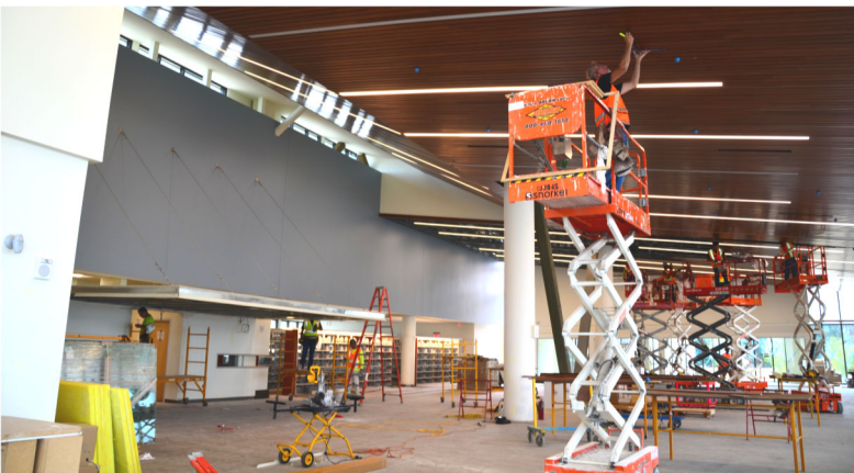
Building 3: Reading room with rulon (linear wood) ceiling
