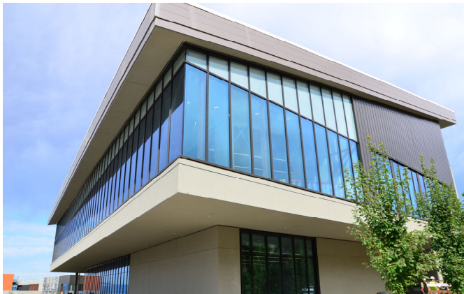
Building 3: Library, southeast elevation
