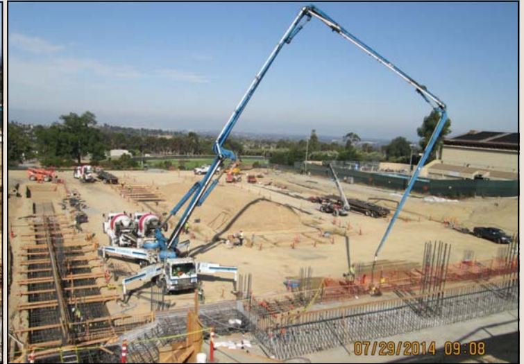
Concrete Pump Truck for Footing Placement
