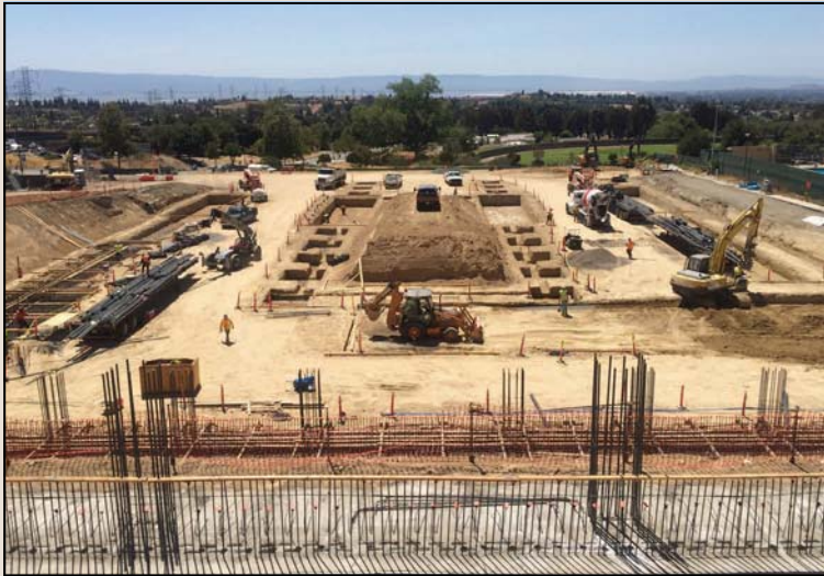
Rebar Placement for Parking Structure Footings
